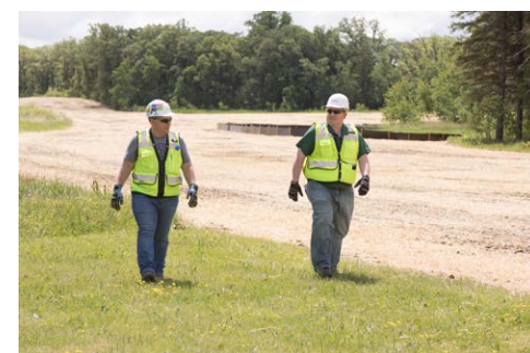
> Every day, replacement of Line 3 is moving closer to completion, shifting focus to restoration of the right of way. Near Thief River Falls, MN.
