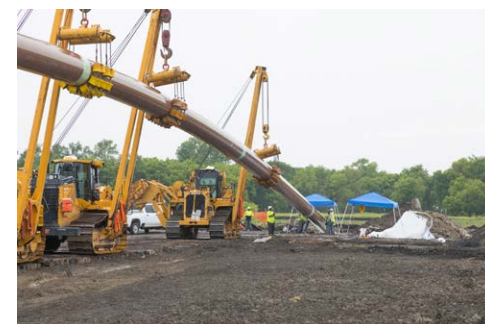
> Horizontal direction drilling is a technique used to minimize impacts to the environment and community by drilling under an identified waterway or designated area. All 19 HDDs have been completed. Photo near Thief River Falls, MN.
