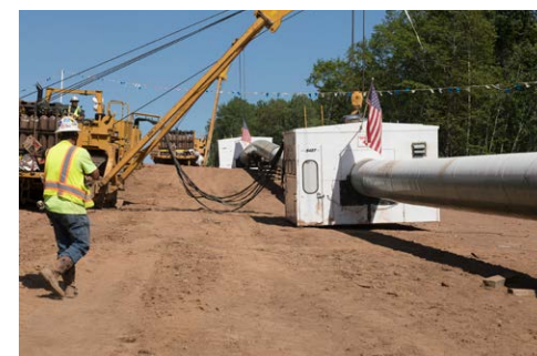
> Pipe sections are welded together, inspected and coated in July near Wrenshall, MN.
