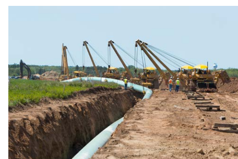
> A section of pipeline is carefully lowered into the trench by skilled union operators. Near Wrenshall, MN.
