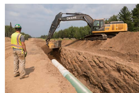
> Soil is carefully placed over the pipeline. As of August 5, more than 330 miles of replacement pipeline is in the ground. Carlton, MN.
