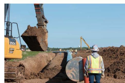
> A trench is dug where the pipeline will rest three to five feet below grade when soil is replaced. Near Wrenshall, MN.
