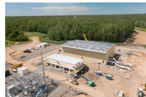
> Temporary work tents are replaced with final building structures housing the pumps that will eventually keep oil flow moving at about walking pace 24 hours a day. Gowan, MN.
